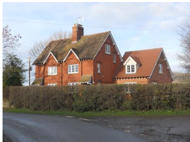
Frampton Farm Cottages
